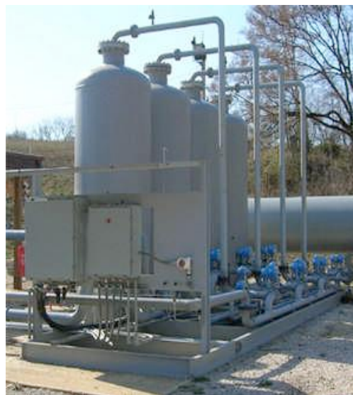
Figure 17: Natural gas treatment unit
