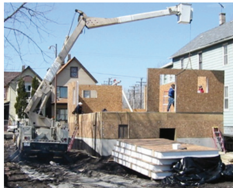
Fig 5: SIP walls being set on a small home
